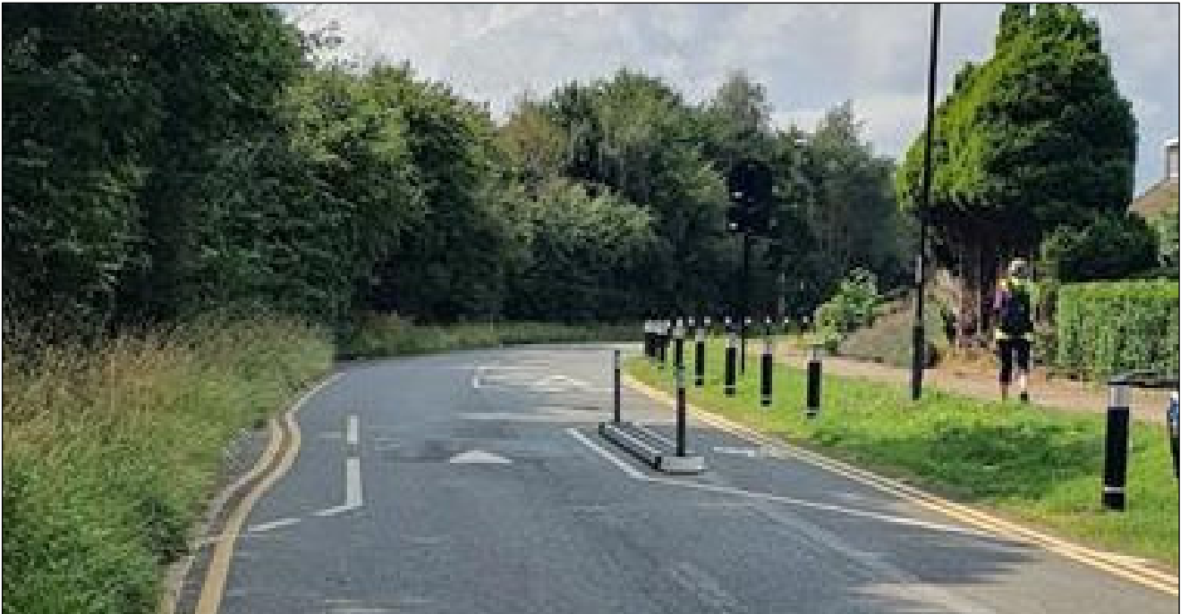
Figure 5-4: Priority Feature with Cycle Bypass
